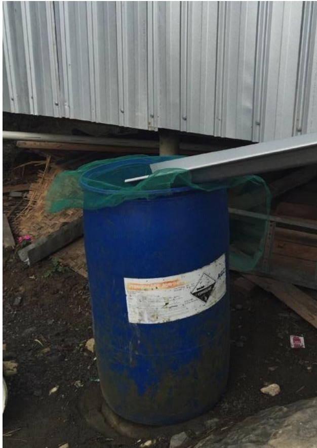
Photo 8 (above, left): One family has tried to improvise a screen to keep debris out of their blue barrel.
